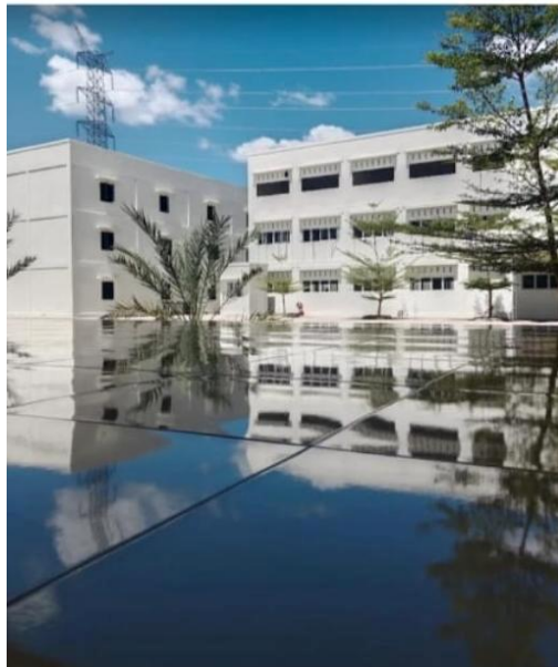
Picture 3. Rear View of The School
